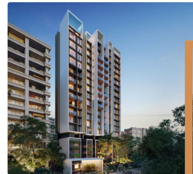
↑ Rustomjee Parishram PALI HILL, BANDRA → SP
