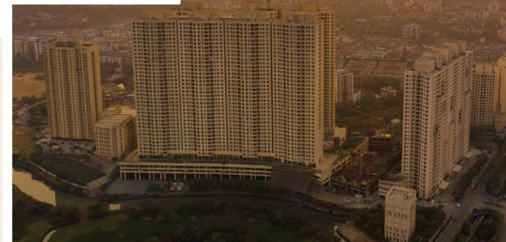
Shot at location - Rustomjee Urbania
