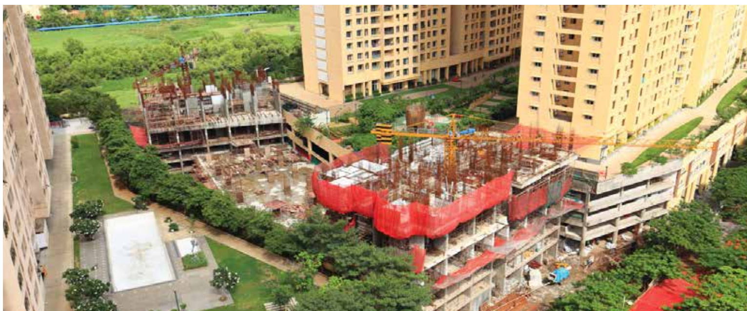
AZZIANO D TOWER: 1ST FLOOR, RCC WIP
