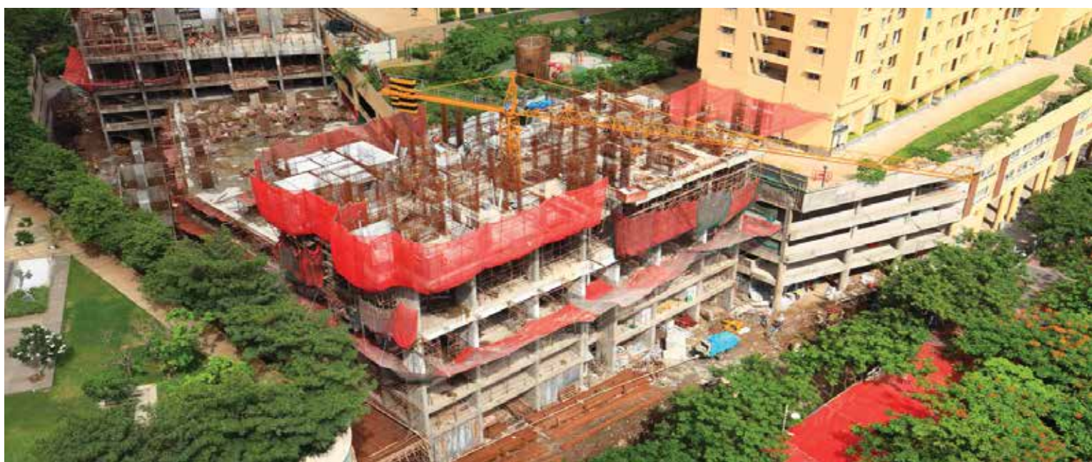
AZZIANO L TOWER: 2ND FLOOR, RCC WIP
